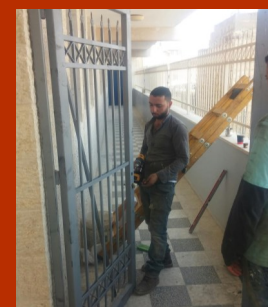
Installation of metal doors to create an additional classroom
