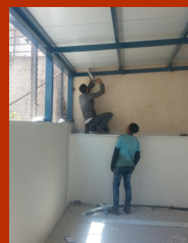
Construction works and covering of the halls
